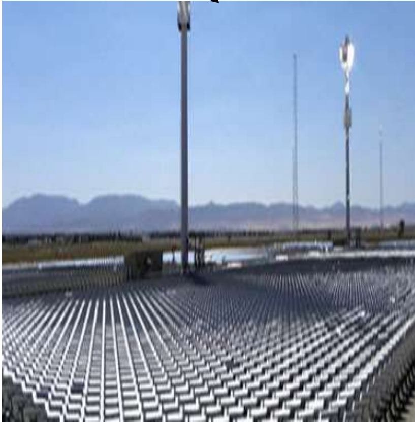
Solar power tower 110 MW
